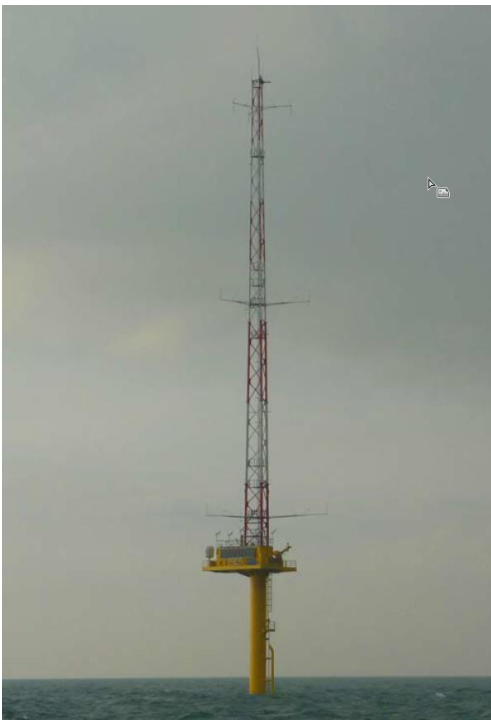
Figure B.1 The offshore meteorological station
