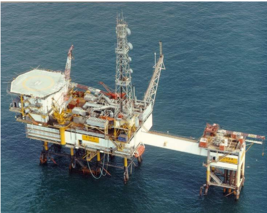
Figure B.8 Aerial view of K13-A platform
