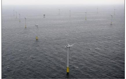
Figure 7-2 Monopiles with wind turbines (OWF Luchterduinen)
