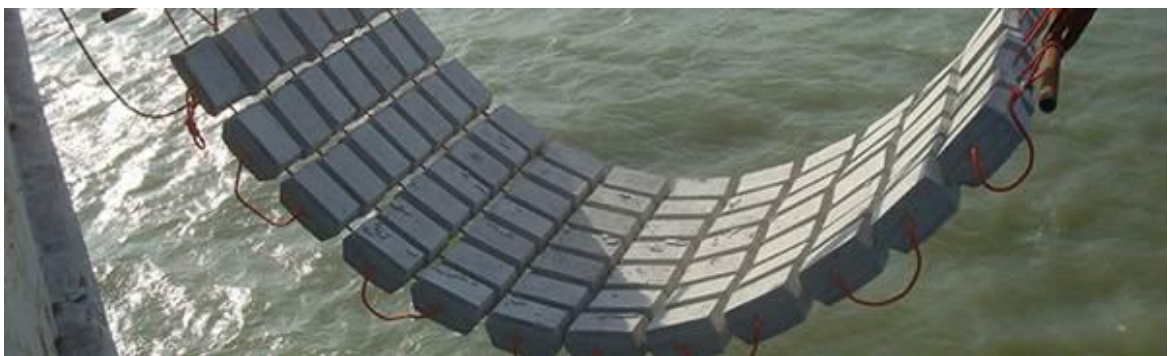
Figure 5.8 Example of a full scale block mattress.
