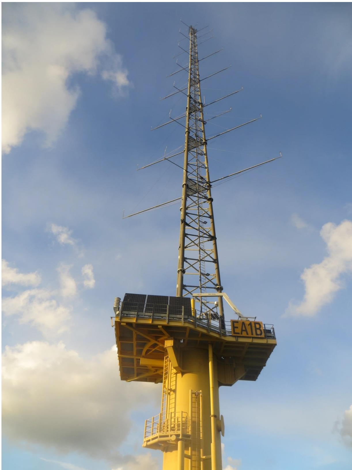
Figure B.3: View of Mast EA1B
