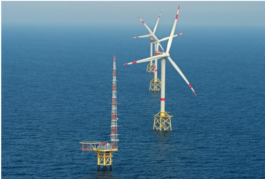
Figure 2-7. Installed FINO 1 met mast [Source: Martina Nolte 4 ]
