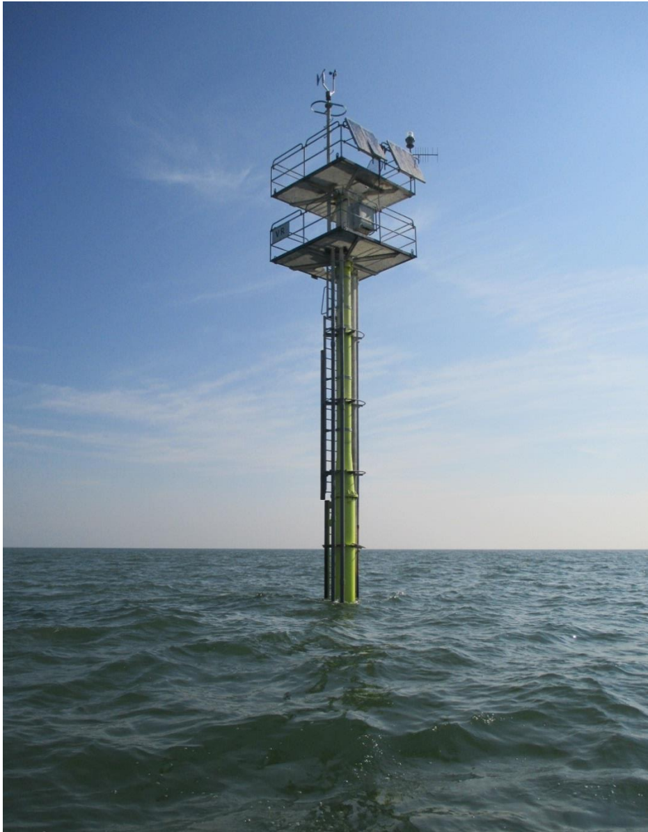
Figure 3.2 The wind measuring station at Vlake van de Raan.
