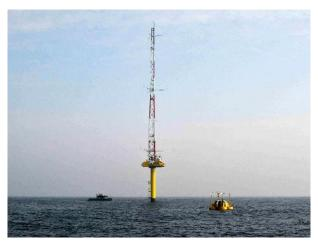
Figure 6 – MMIJ mast (the floating LiDAR next to the mast is being tested and is not included in this study) [source: RWE Innogy]
