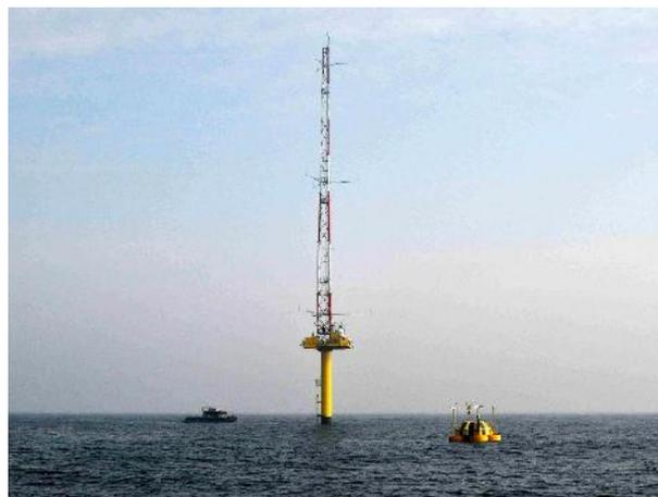
Figure 6 – MMIJ mast (the floating LiDAR next to the mast is being tested and is not included in this study)
