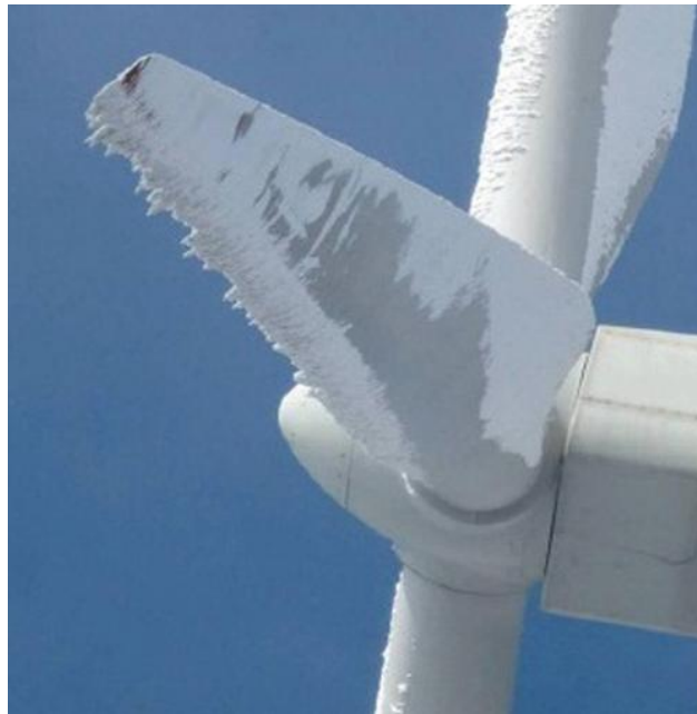
Figure 8.1 Ice accumulation on a wind turbine blade (Source: http://www.windpowerengineering.com ).
